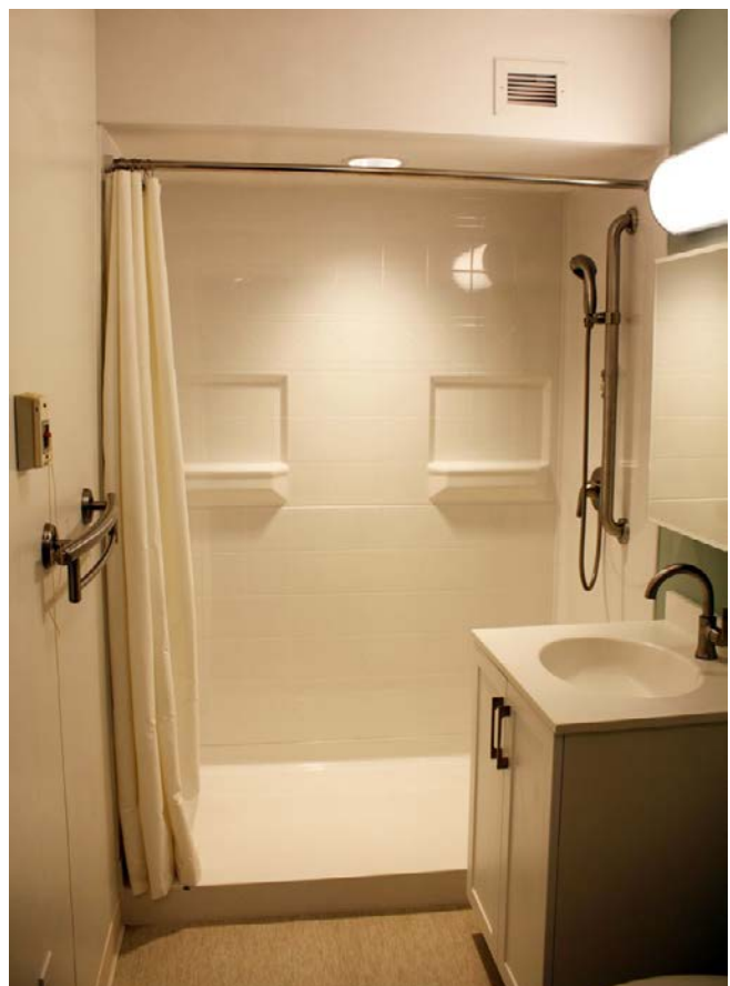
Top: Bathroom large enough to accommodate an aide. Bottom: Install showers in all units; task lighting in shower and over vanity.
